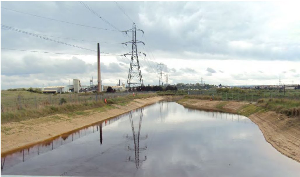
Figure A12 The lagoon at TN23 with steep-sided bare soil banks. The water is discoloured red/brown- possibly due to leachate contamination
